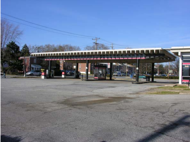
Canopy that previously covered gas pumps
